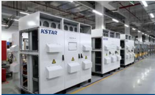
PV Assembly Workshop
